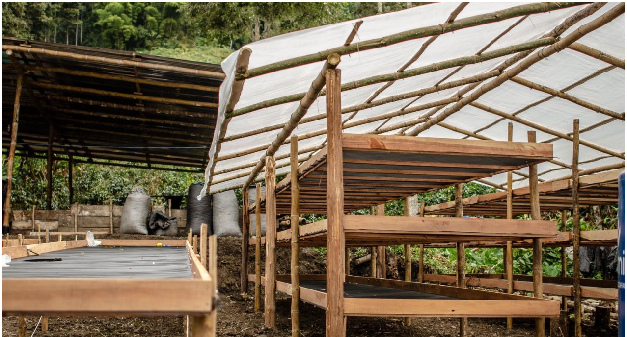
Fig.1 Example of covered drying beds constructed
